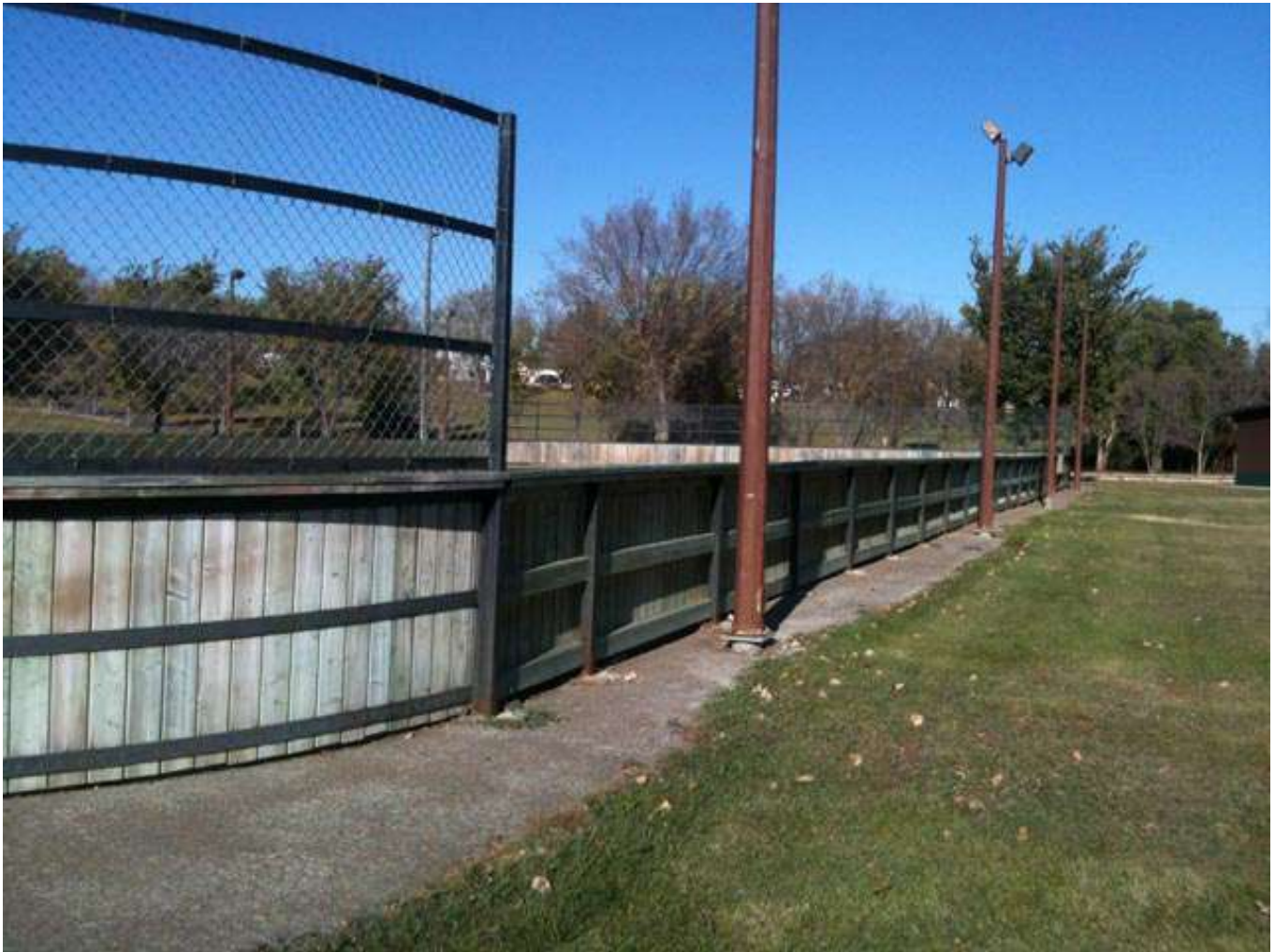
An example of an outdoor ice rink, in Swift Current, Sk, Canada, that incorporates weathering steel posts, wood boards, and a wire mesh framework on the south side.
