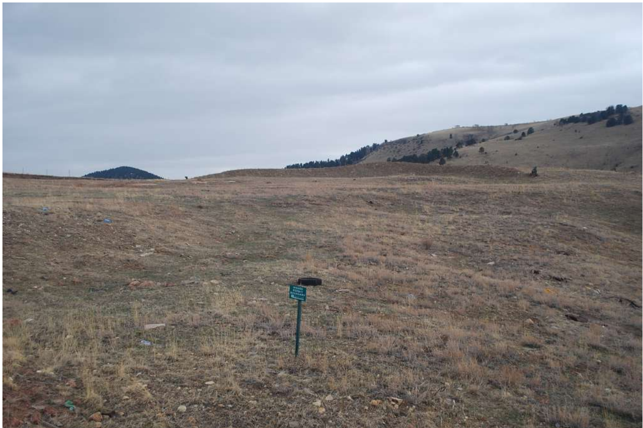
The old landfill has been capped with soil and revegetated. This is a view of current conditions, looking south east across the site. There is broken glass that needs to be cleaned up at the surface.
